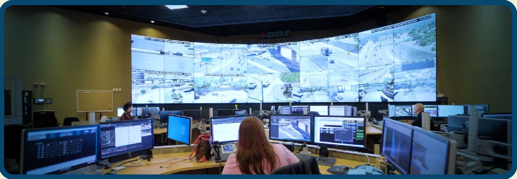
The ADOT Traffic Operations Center will monitor the flex lanes with cameras and will control the gates and VAB remotely.
