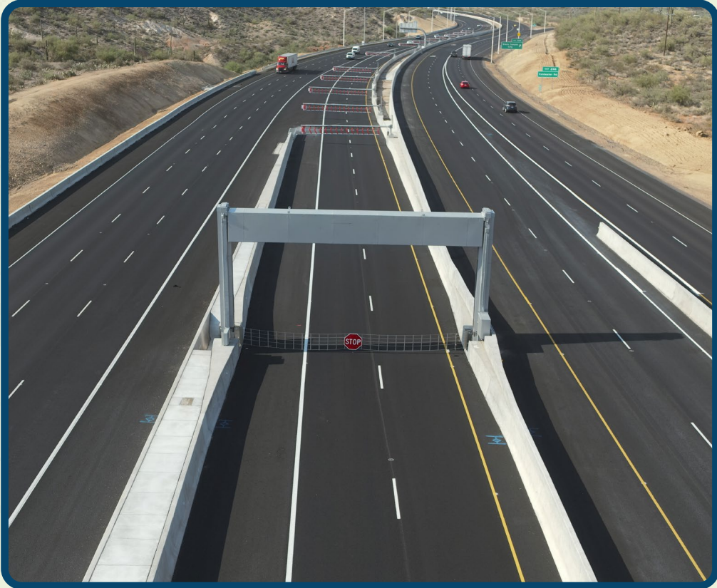
A specialized, automated Vehicle Arresting Barrier (VAB) is located at both ends of the flex lanes and will be used to prevent vehicles from entering the flex lanes when traffic is flowing in the opposite direction.
