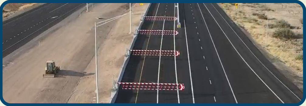
Automated swinging arm gates on both sides of the VAB will extend when the flex lanes are closed to a direction of traffic, blocking the entrances to the lanes and indicating to drivers that the flex lanes are closed in the direction they're traveling.
