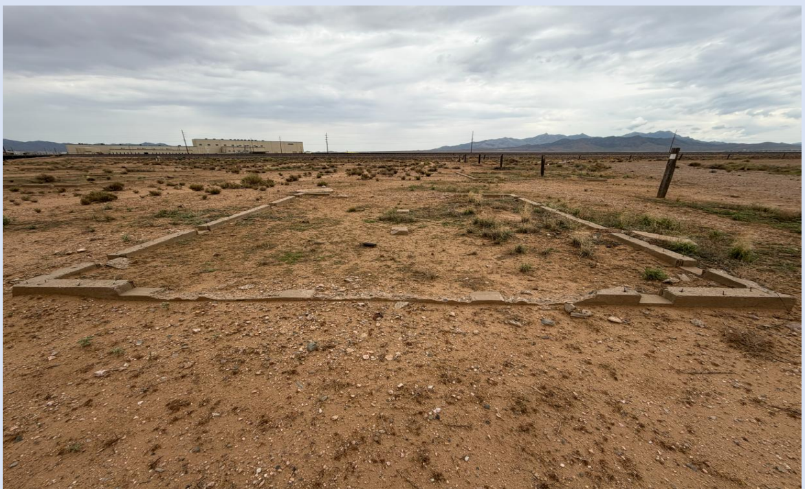
PHOTO 8: TYPICAL CONCRETE WALL BASE
