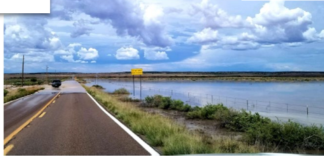
Roadway overtopping at around Sta. 432+00 South of Existing Box Culvert.
