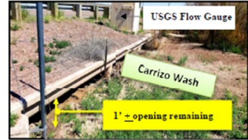
Photo 1: Siltation at Inlet of Existing 6 - 10'X8' CBC located at Carrizo Wash, MP 323.85
