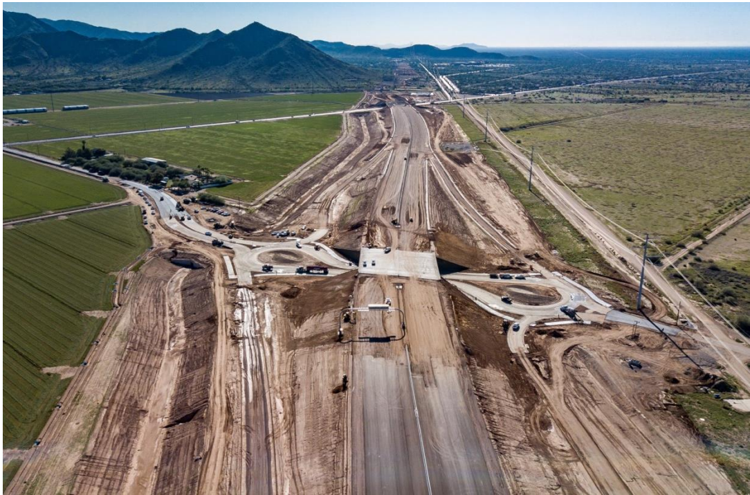
South Mountain Freeway
