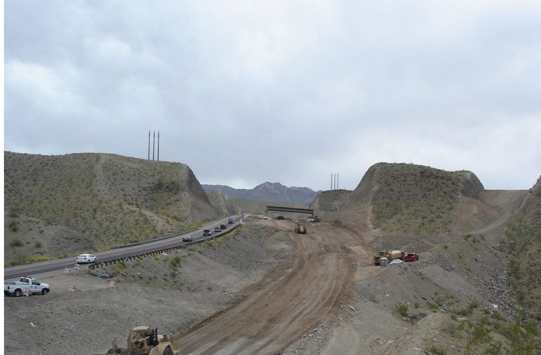
US 93 Two Lanes to Four Lanes
