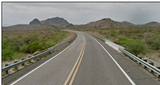
Figure 19: Slick Rock Wash Bridge #2
