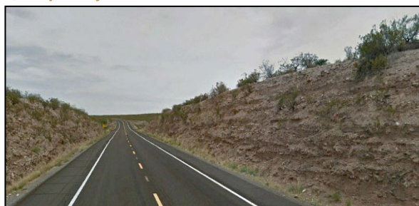
Medium/Major: higher slope/rock cut
