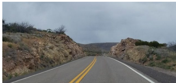
Figure 15: Rock Cuts Adjacent to Edge of Pavement
