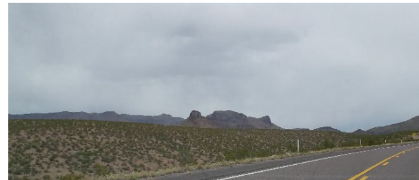
Figure 13: Steep Embankment with No Guardrail Protection
