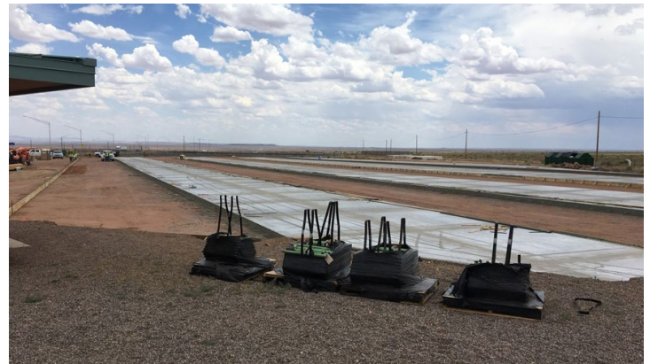
Credit: Arizona Department of Transportation
