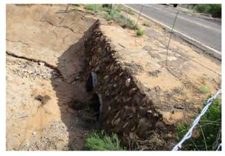
Figure 188: CMP outlet with concrete protection facing northwest
