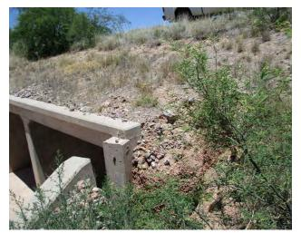
Figure 173: Outlet Box Culvert Wingwall Erosion
