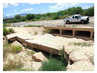
Figure 162: Pomerene Rd. Box Culvert is Broken at Both Edges of the Inlet
