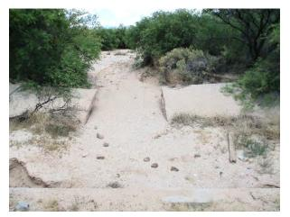
Figure 158: Ramsey Rd. Outlet at Box Culvert, Annual Sediment Overflow
