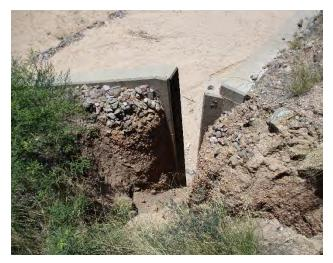
Figure 172: Outlet Box Culvert Wingwall Erosion
