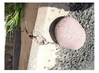
Figure 163: Pomerene Rd. Box Culvert is Broken at Both Edges of the Inlet
