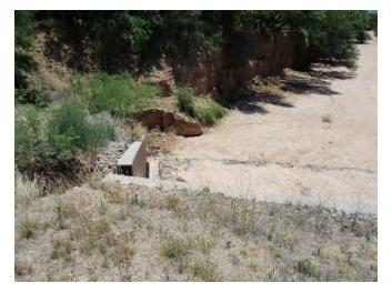
Figure 174: Outlet Box Culvert Wingwall Erosion
