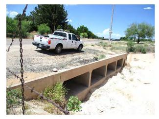
Figure 160: Pomerene Rd. Box Culvert Inlet Overflow
