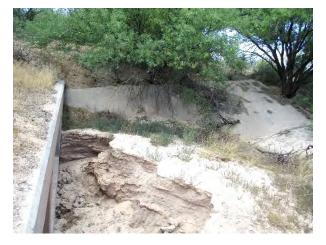
Figure 157: Ramsey Rd. Inlet Dike Failure, Box Culvert Too Small for Water Flow
