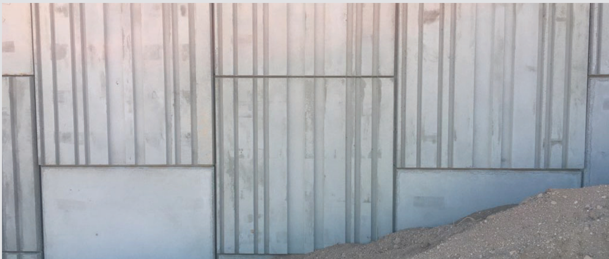
Panels on Wing Wall with Random Vertical Rustication Pattern
