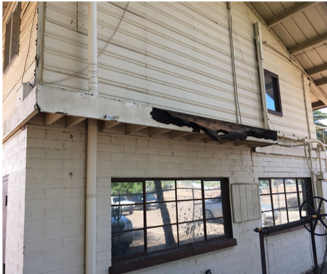
Damaged/rotting wood at the exterior
