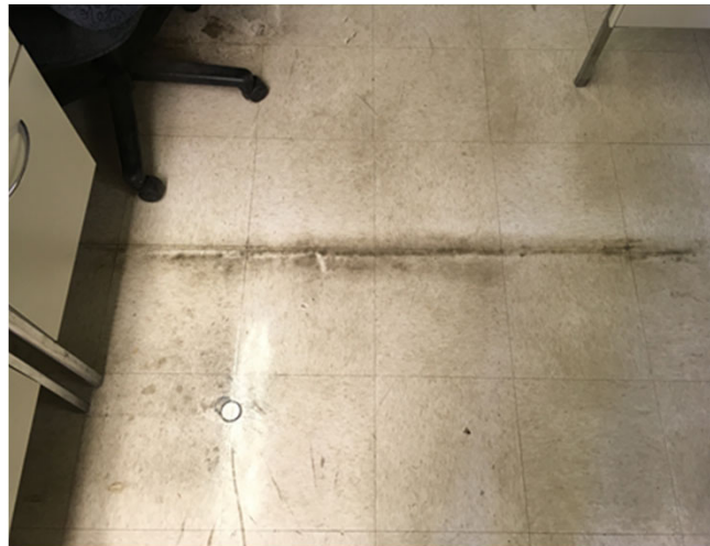
Water damage on the floor tiles
