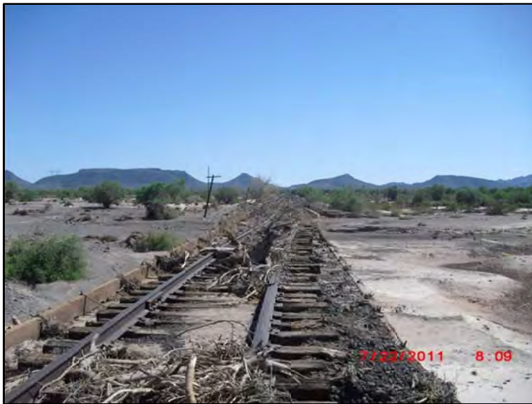
Photo 3: Washout at Milepost 842.75 (Photo provided by UPRR)
