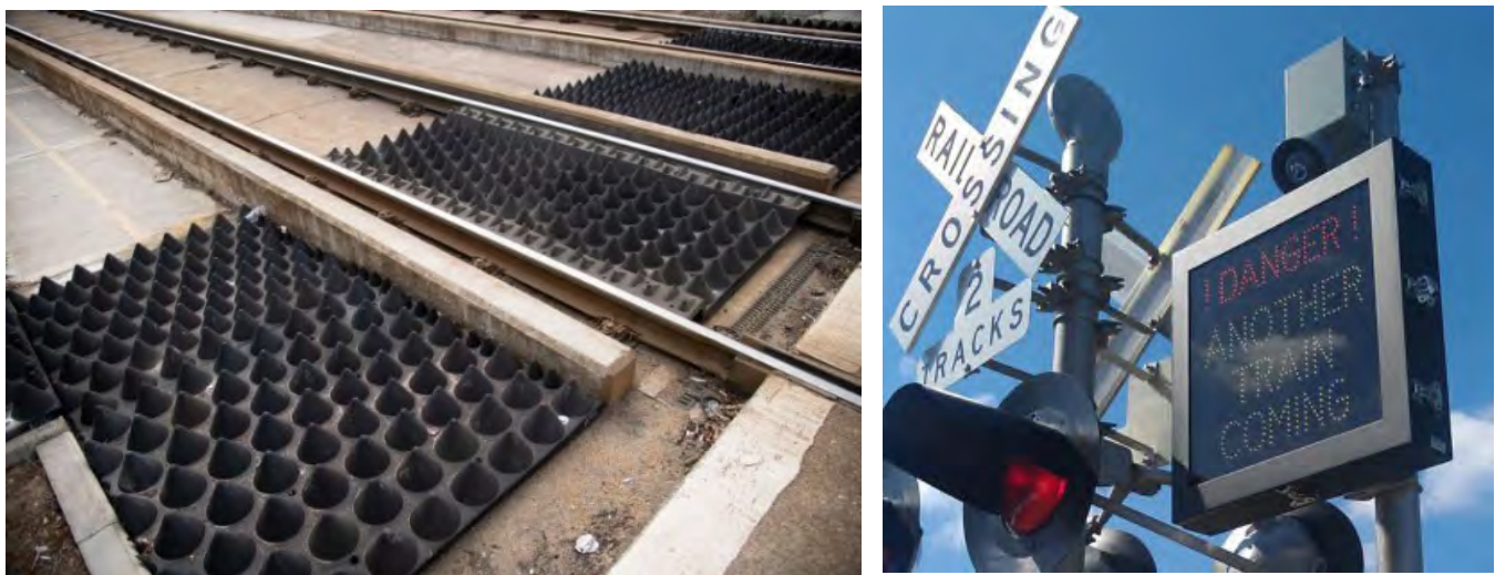
Figure J-3: Conical Trespasser Matting and 'Another Train Coming' Warning Sign
