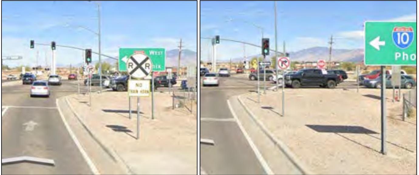
Figure 4: “Sign Clutter” Eastbound; Visibility Obstructed
