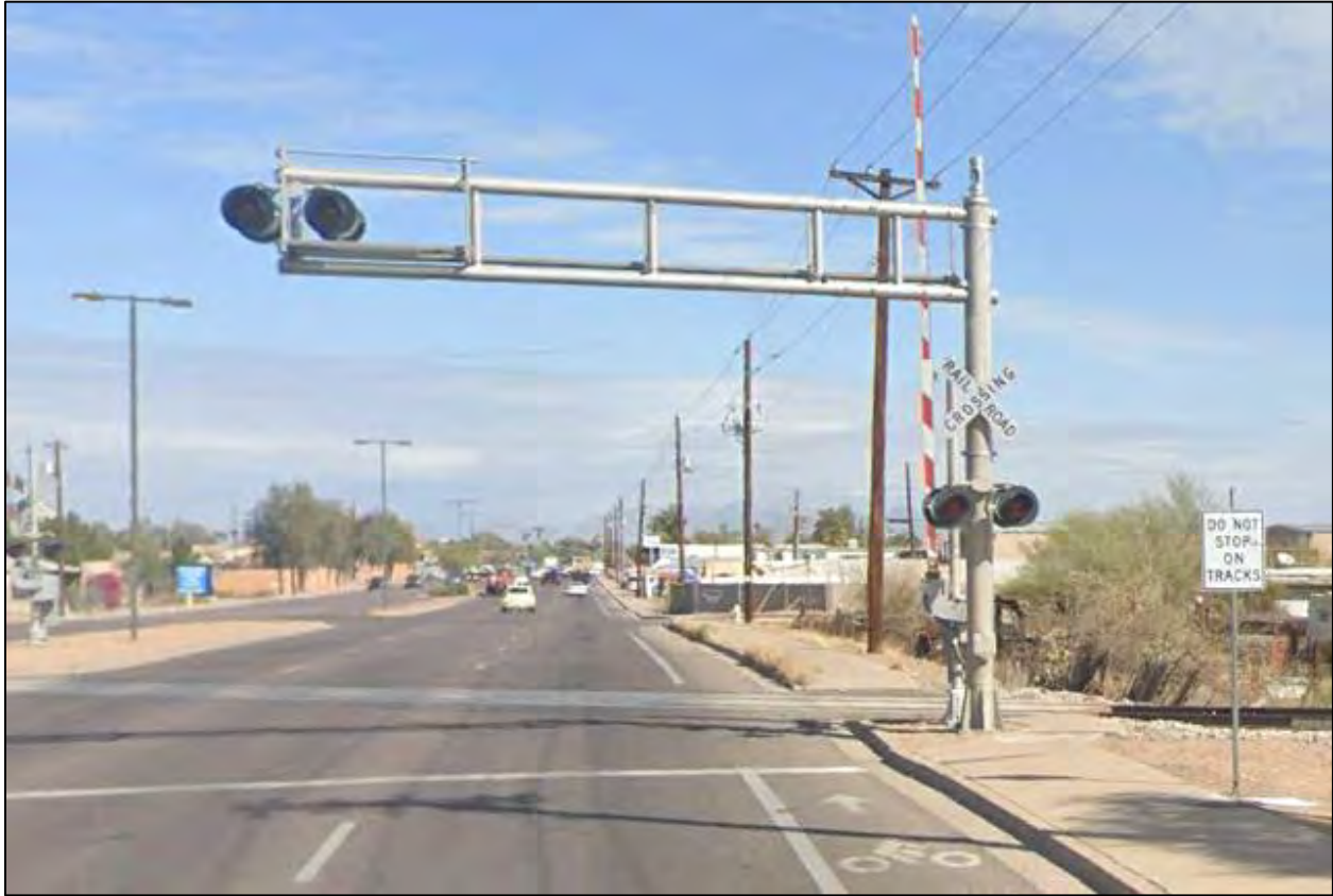
Figure 2: Limited Pedestrian/Bicycle Warning Devices
