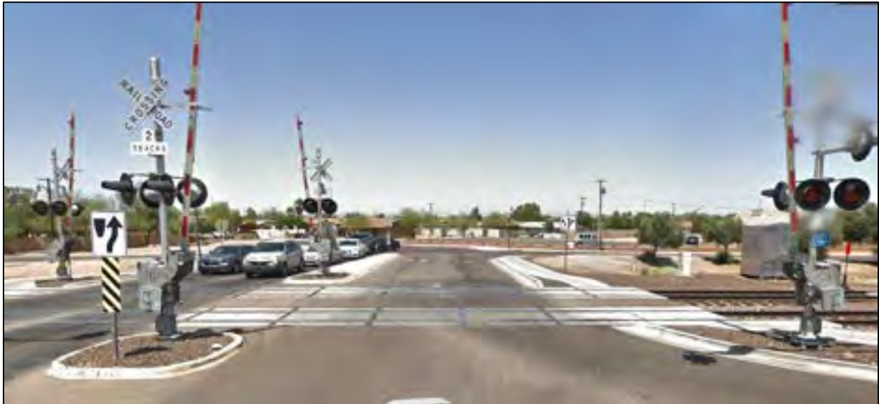
Figure 1: Flashers and Gates, Faded or Missing Pavement Markings
