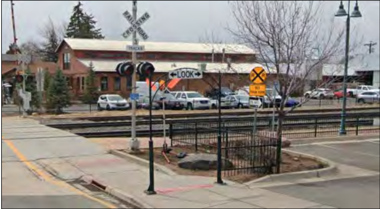
Figure 2: Pedestrian Signage and Fencing
