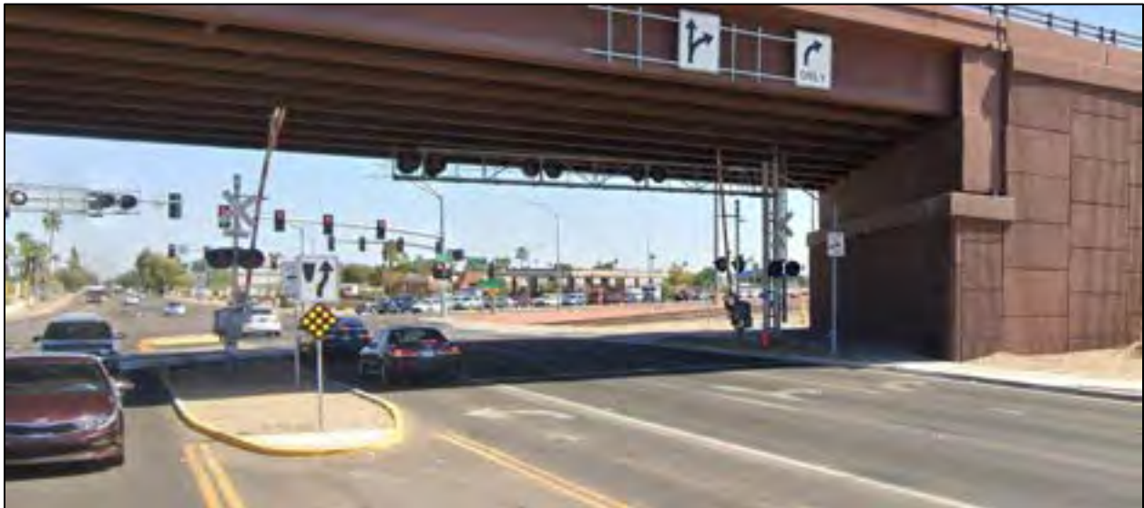
Figure 1: Shadow Reduces Visibility of Gates
