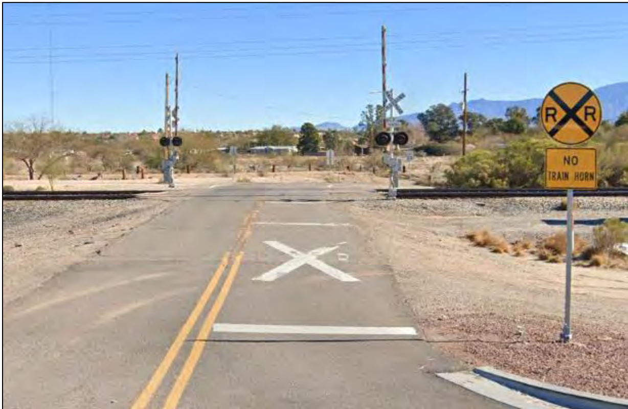
Figure 1: Existing Flashers and Gates
