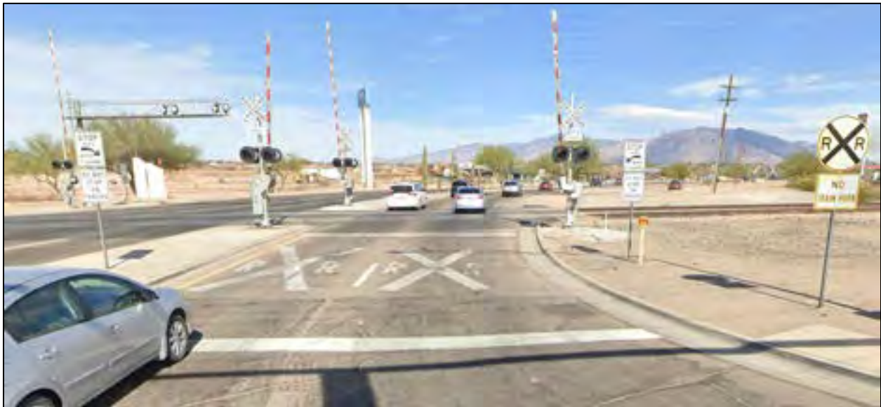
Figure 1: Street-Level View Eastbound - Flashers and Gates
